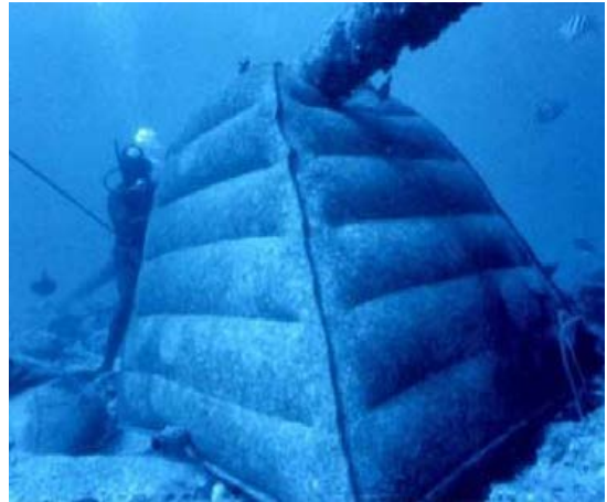
Figure 2: Basic details for grout bag span correction for higher height correction
