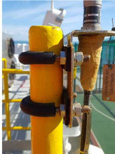
Figure 2: Insulation to avoid galvanic corrosion.
