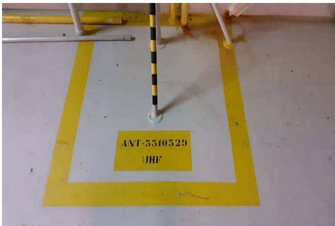
Figures 6A and 6B: Examples of antenna's identification on the floor.
