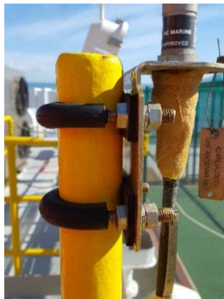
Figure 2 – Example of cable fixing
