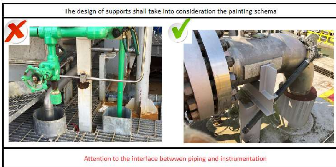
Figure 15 – Carefully with piping and instrumentation interface
