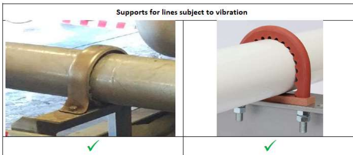
Figure 14 – Other example of solutions for lines subjected to vibration
