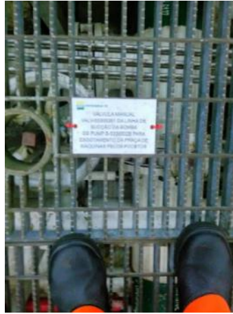
Figure 20. TAGs on floor gratings
