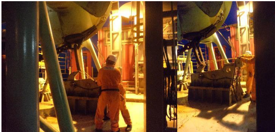
Figure 16. Secondary maneuver for connecting the hawser to the emergency device
