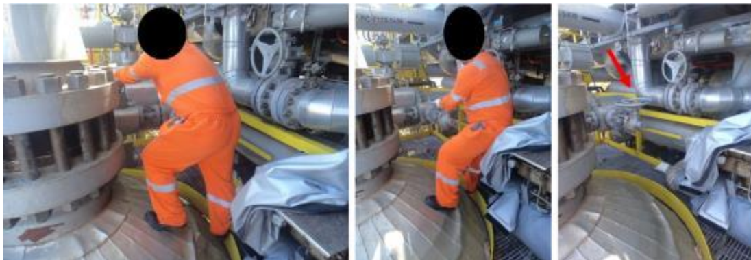
Figure 5. Irregular surface (top of vessel) to valve access support.
