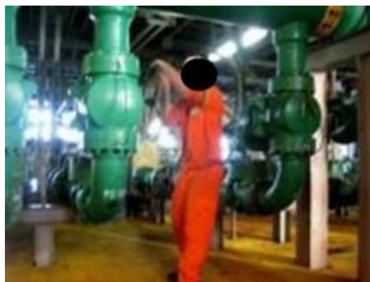
Figure 16. Handwheel position, allowing the use of body weight as support.
