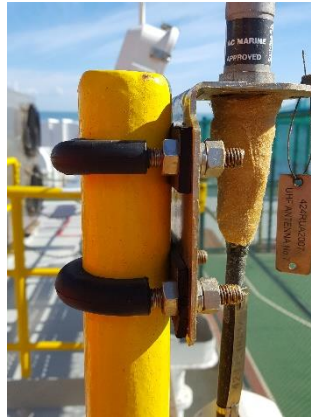
Figure 1: Example of installation to avoid galvanic corrosion
