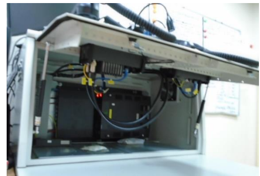
Figures 8A and 8B: Example of easy access to equipment rear inside the console.
