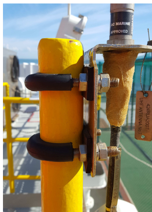
Figure 2: Example of installation to avoid galvanic corrosion.
